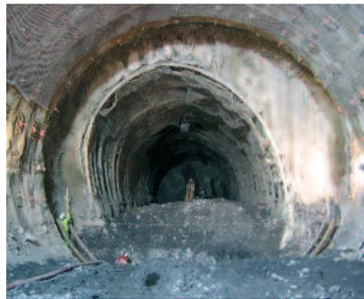
rock mass. Exceptional convergences, of more than 2m in diameter, caused tunnel linings to rupture and the tunnel advance to slow to a virtual standstill.
